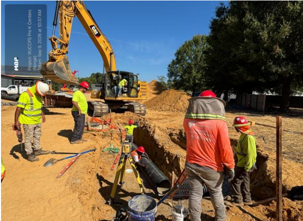
Toano: Tie in storm water structure
