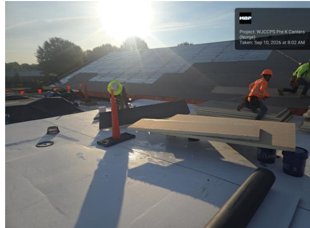
Eastern: Installing insulation and watershed on sloped roof (Section A)
