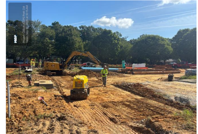
Toano: Grading and compacting parking lot area
