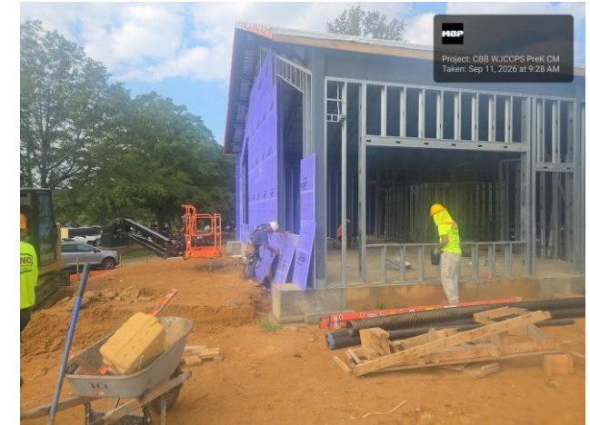
PD Interiors: Installing exterior sheathing (Section A)
