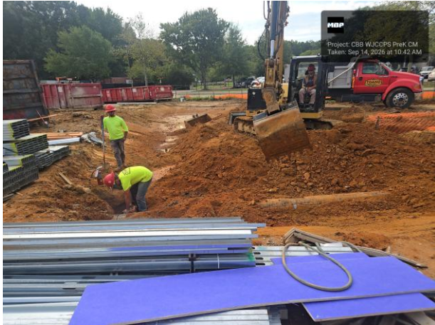
Toano: Excavating storm basin B
